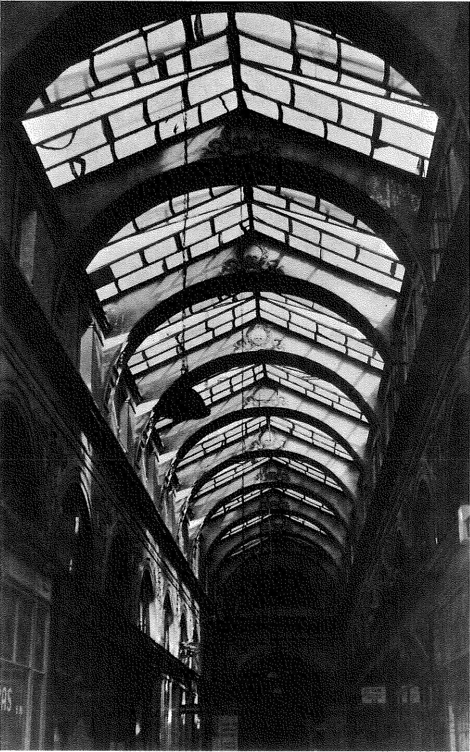
Glass roof and iron girders, Passage Vivienne. Photographer unknown. Collection of Johann Friedrich Geist; courtesy Prestel Verlag, Munich. See A1a,2.
