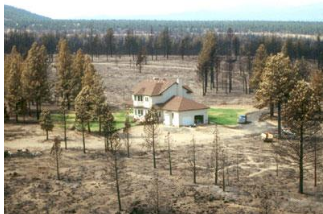
Home surrounded by wildland that survived a fire due to good defensible space.
