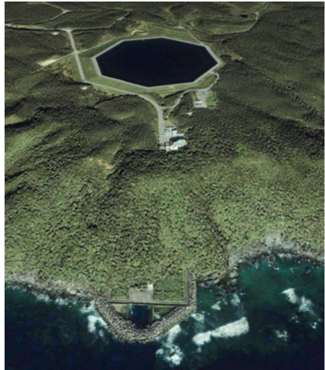
Pumped hydro storage using seawater in Okinawa
