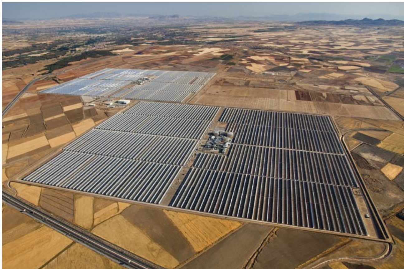
ACS Cobra Energia's Andasol 1 & 2 solar thermal with storage plants in operation in Granada, Spain 63 .
