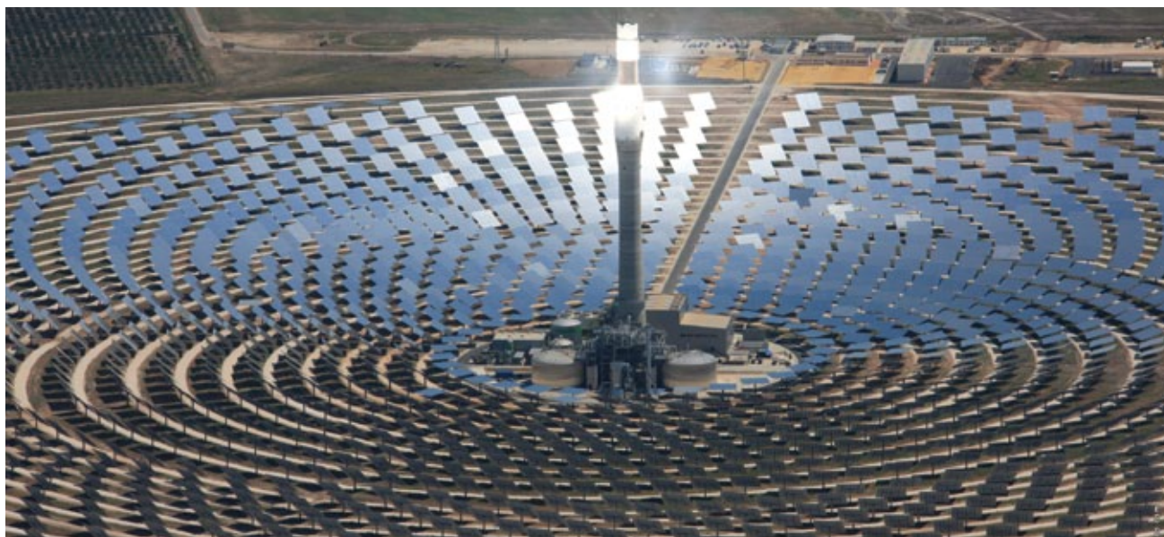
Torresol Gemasolar solar thermal power tower, Spain SOURCE: TORRESOL
