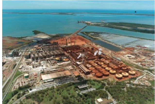
Queensland Alumina Refinery at Gladstone 128 .
