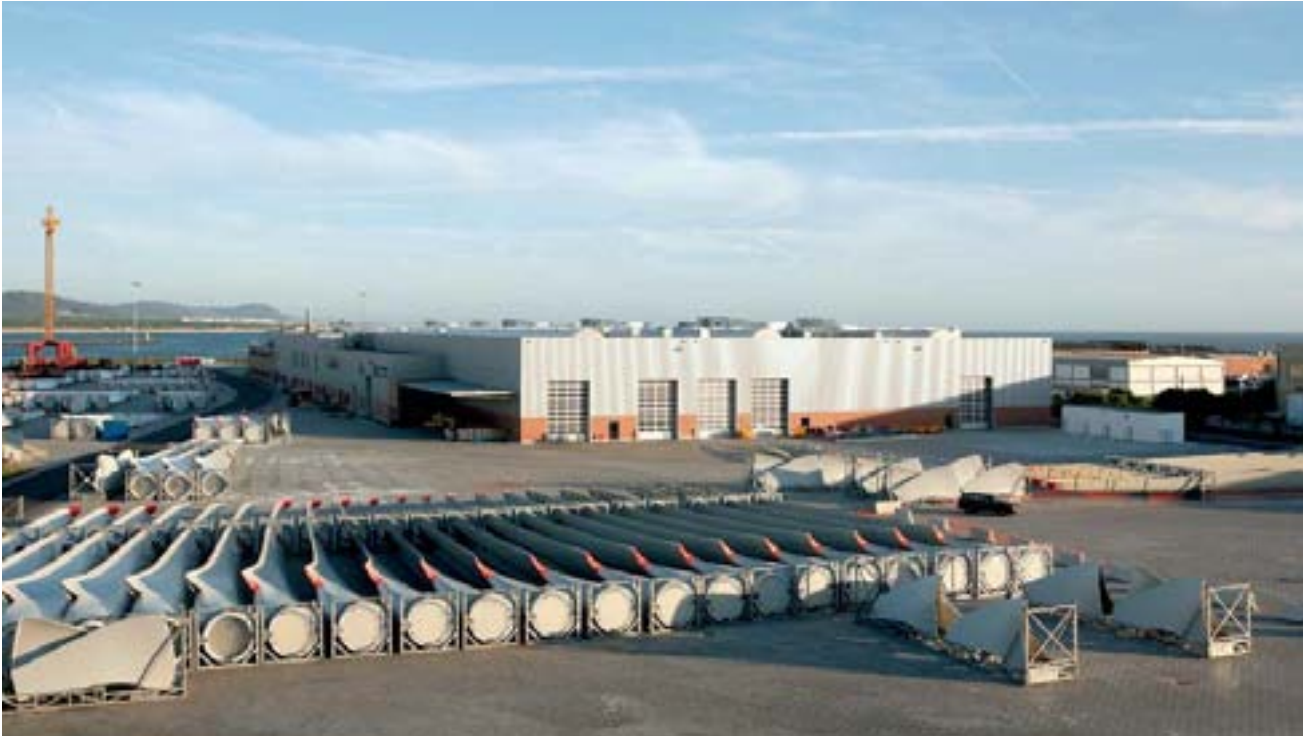
Enercon rotor blade factory in Viana do Castelo, Portugal 31
