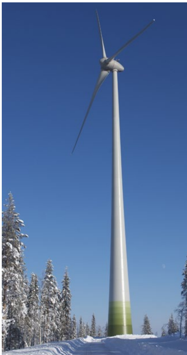
Enercon Wind Turbine, Sweden 104
