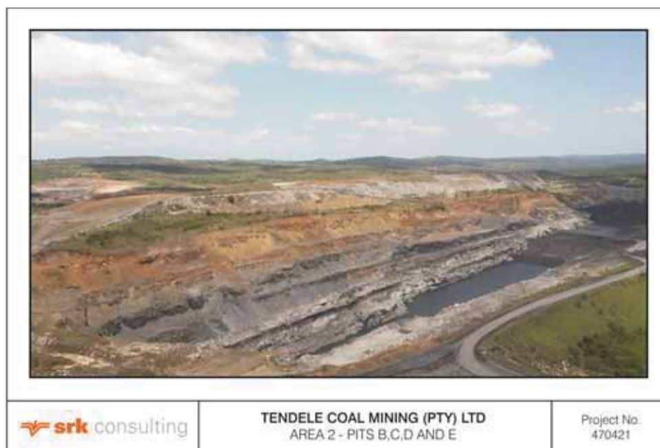
Figure 5-1: Area 2, Pits B, C, D and E
